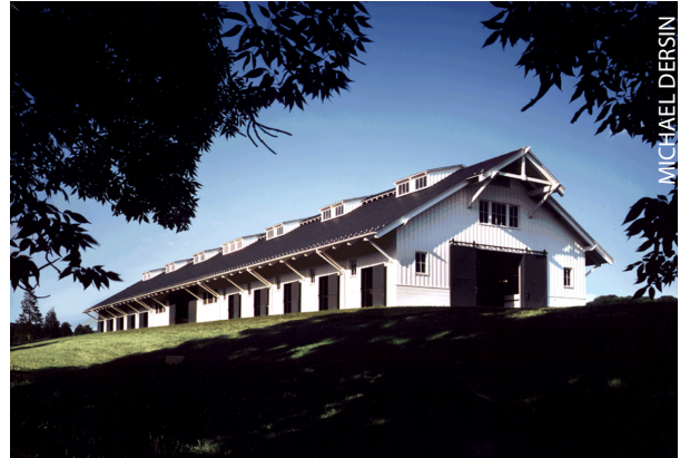
Morven Stud in Charlottesville, Virginia, sits atop a hill positioned to catch prevailing breezes.
