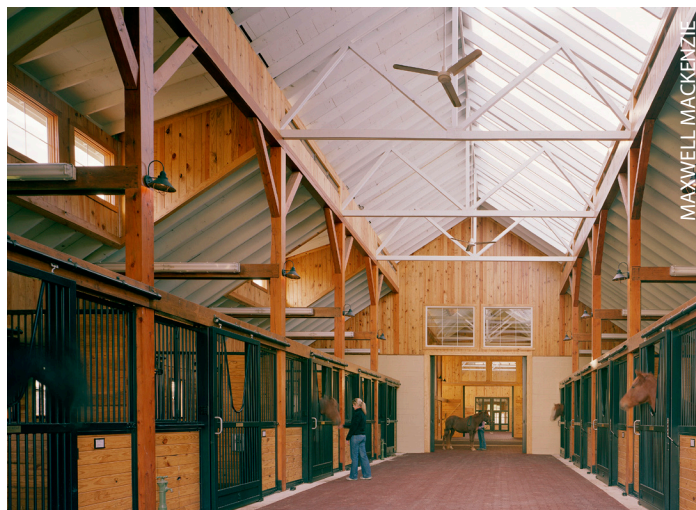
The passive lighting and ventilation designed into this Virginia stable using skylights and ridge vents reduces the risk of both fire and disease.
