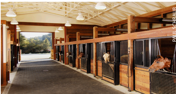
This Northern California barn is built with wide aisles and horse-friendly materials such as interlocking rubber brick flooring and smooth metal yoke gates for safety and comfort.
