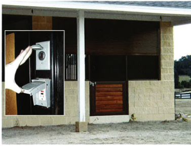
Explosion-proof outlet covers and roll-down hurricane gates are some options for mitigating the risk to your barn posed by fire and wind damage, respectively.
