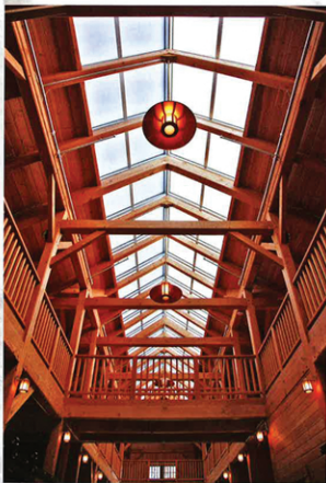
Skylights can reduce the need for electric lights and box fans, reducing risk of electrical fire.
