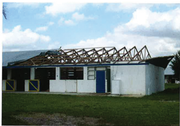
Gabled roofs can take a beating during hurricanes, and must be reinforced with braces.
