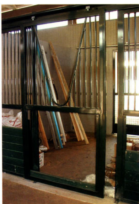
Powder-coated stall fronts are more common today allowing barn owners to spruce up with color.
