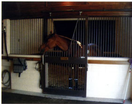
Make sure bars are no more than two inches apart or use a mesh design to avoid hoof injury. Full-view doors make checking in on horses much easier.
