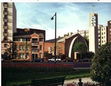
The new rectory abuts the 1961 Church of St. Stephen Martyr.
