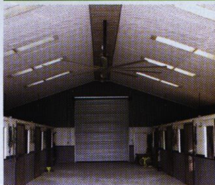
Left: This barn aisle uses a Big Ass Fan to improve ventilation year round and to help keep the barn cooler in the summer. Middle: The Equustall system uses interlocking panels filled with drainage material to keep stalls dry. Right: The Stable Grazer allows for easy feeding and less mess on the stall floor.
