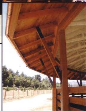
The 60' diameter round pen awaits finishing touches; details include deep overhangs of beautiful cedar decking and elegant copper gutters supported by redwood timber outriggers.
