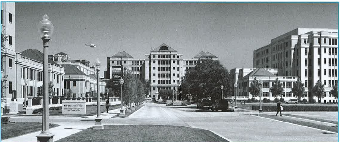
Cook Children's Medical Center expansion in Fort Worth, TX. Photo provided by David M. Schwarz Architects.
